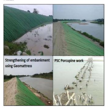
Fig. 7. Implementation of geotextile mattress and porcupine works
