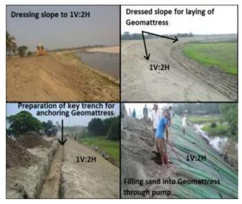
Fig. 5. Installation of Geotextile mattress at various stages
